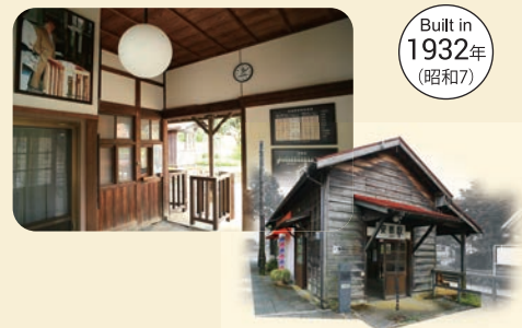
4 安部駅本屋 Abe Station Main Building
