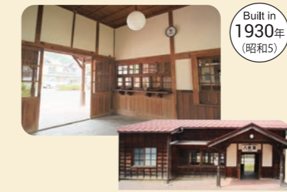
6 八東駅本屋 Hatto Station Main Building
